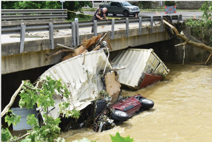
2025 June Flood – Ohio County (photo by Eric Ayres)
